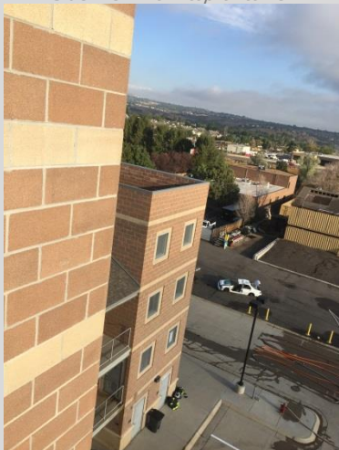
Side View from top of tower
