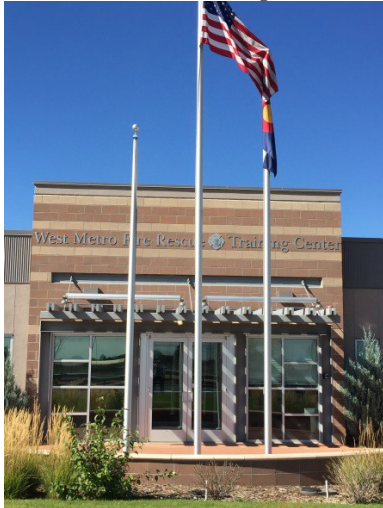
Front of Building
